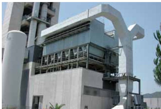
Filter in cement plant
