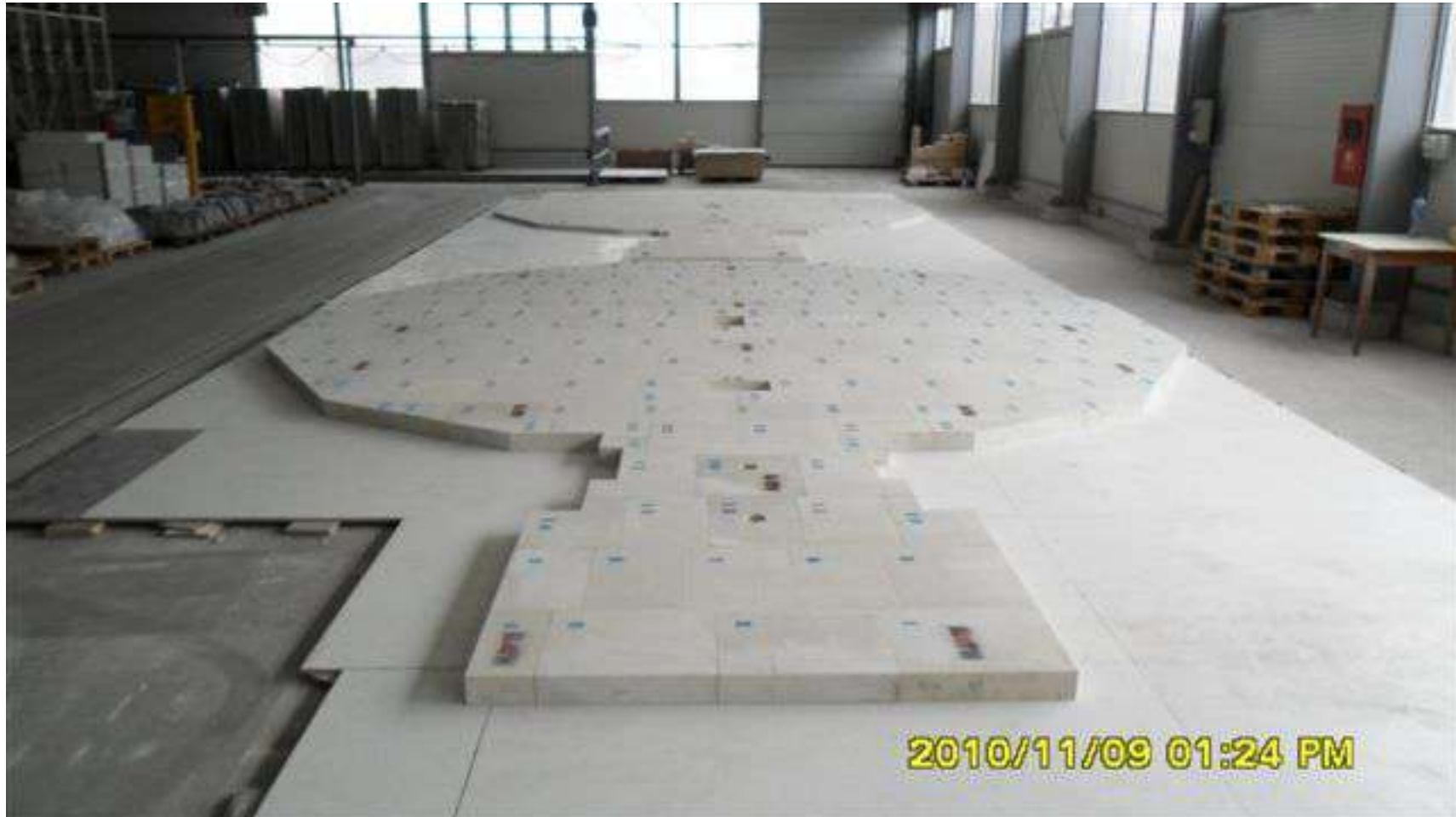
Melting tank bottom layers – tableware furnace
