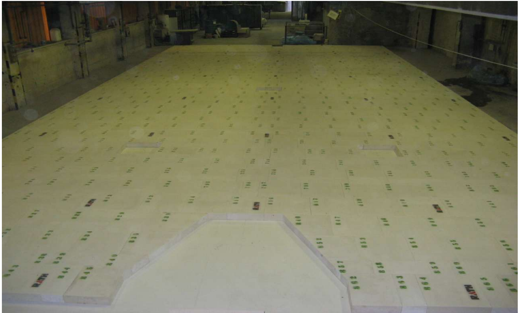
Melting tank – andalusite-mullite bottom from Silrath AK60M
