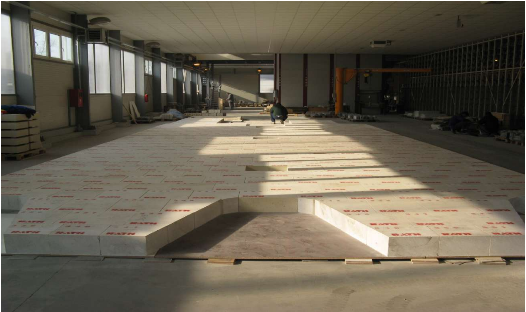
Melting tank – andalusite bottom from Silrath AK60
