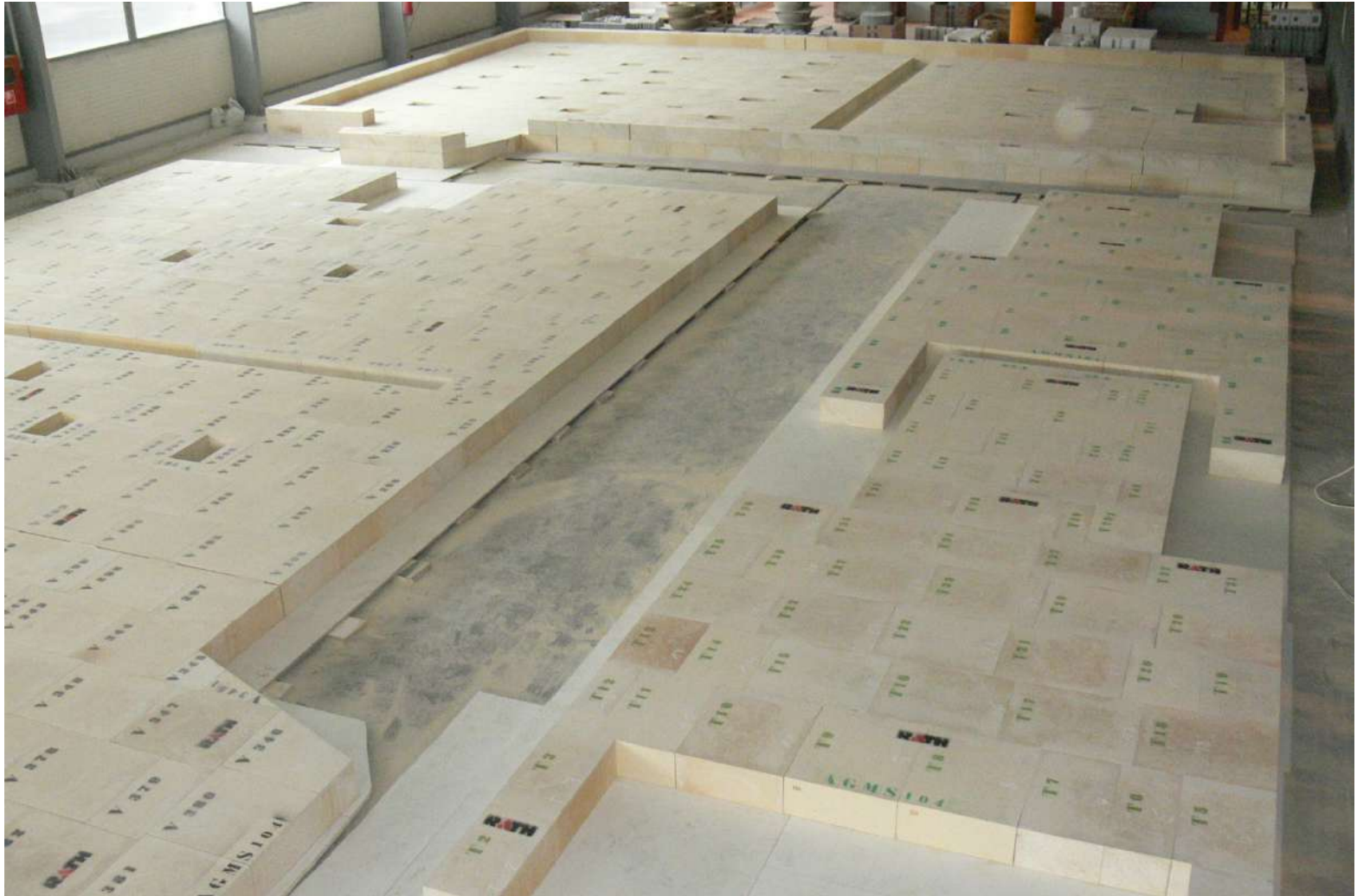
Melting tank, working end – fireclay bottom layer from Suprath T45
