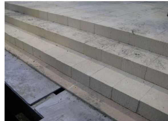
Insulating brick layers – melting end bottom
