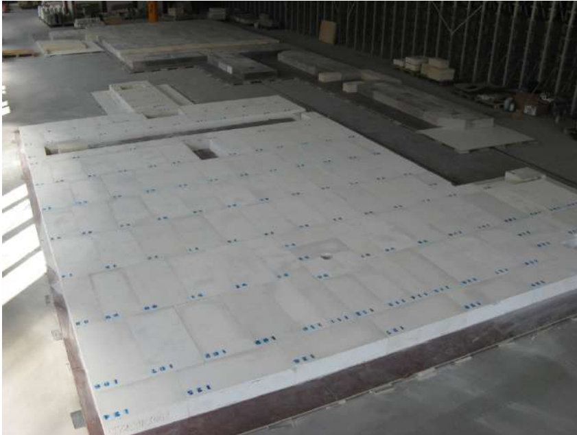
60%- \text{Al}_2\text{O}_3 – Andalusite (Carath 1650LC-SF) and 40% \text{Al}_2\text{O}_3 – Fireclay ME bottom layers (Carath 1360LC)
