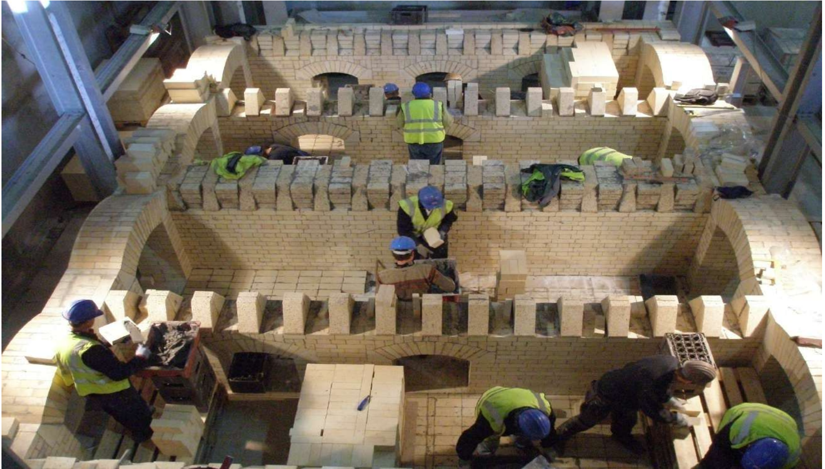
Construction of the fireclay/downpart regenerator – Suprath A40t, Suprath T45
